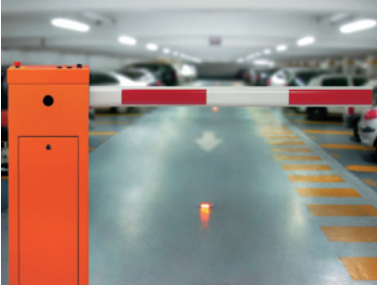
ATV12 controlling an access barrier
