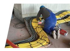
This cable is specially designed to meet standards IEC 60332-3, EN 50266 and NBN C30-004 F2 standards with a fireproof and halogen-free sheath, which does not give off/release toxic or corrosive fumes. Its electrical performance is also certified by an independent third-party body.
