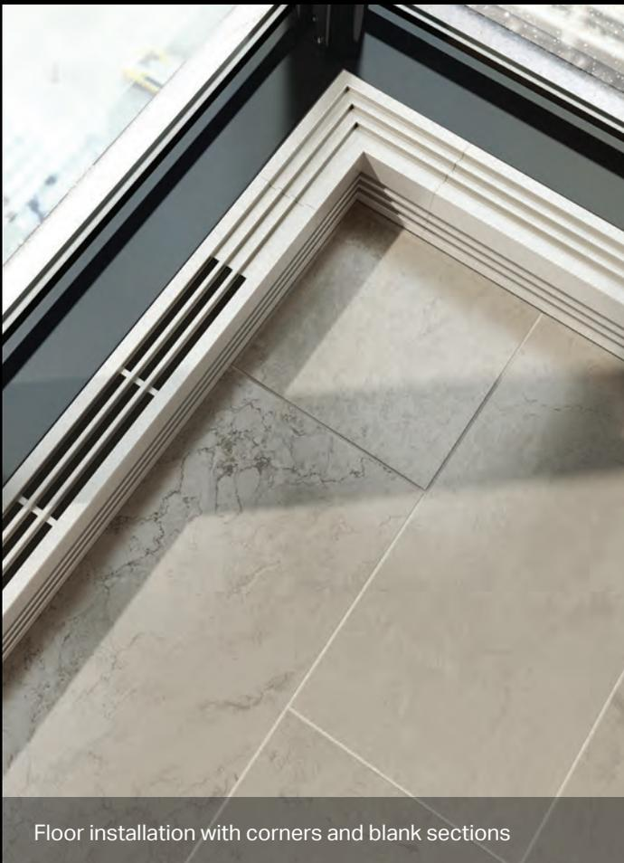
Floor installation with corners and blank sections
